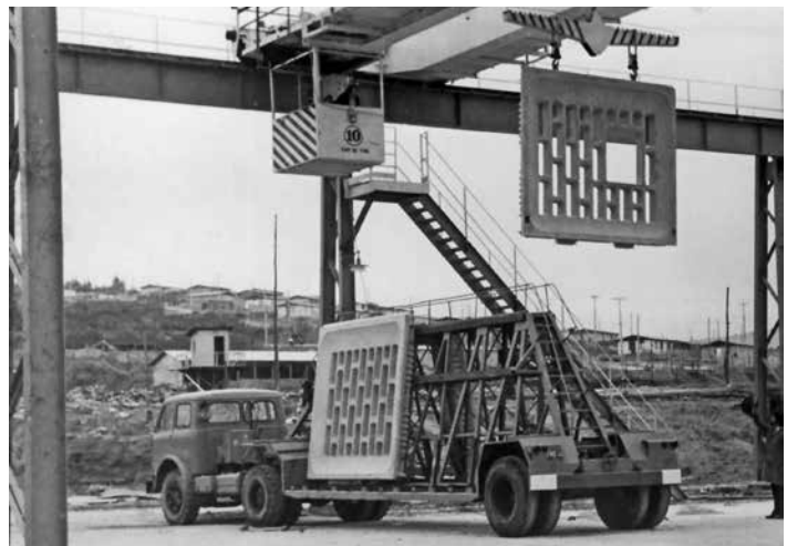
Salida de distintos modelos de paneles perforados, desde la fábrica en dirección a la obra. Quilpué, Chile, c. 1973. Models of perforated panels leaving the factory towards the construction site. Quilpué, Chile, c. 1973. © Norberto Salinas González
