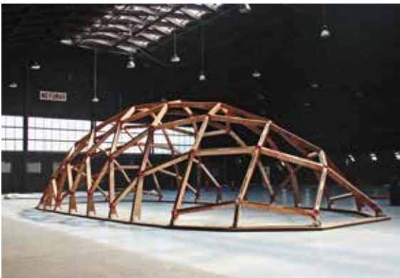
Estructura Torsionoid / Torsionoid structure © Pol Taylor, Marcelo Bernal & Francisco Valdivia
