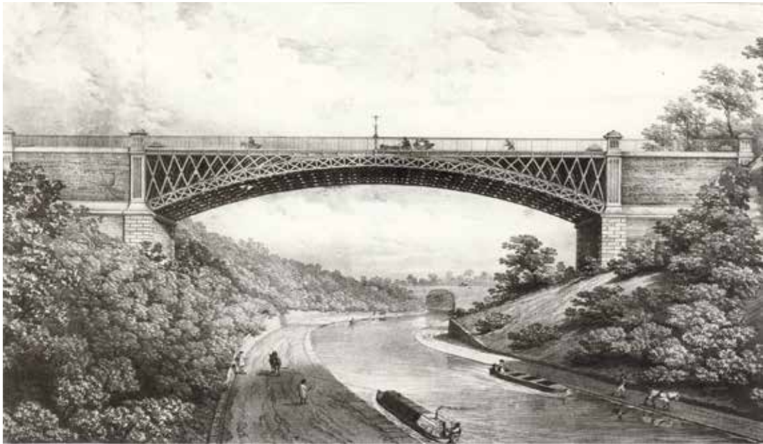
Lámina 2. Las gabarras (“joeyboats”) de Pickford’s pasan por debajo del puente de hierro de Galton, Smethwick. Ingeniero Thomas Telford, 1829. British Waterways Archive, Gloucester, UK (BW192/3/2/2/2/52). “Drawing of Pickfords joey boat and horses at Galton Bridge on the Birmingham Canal Navigations”. Lithography por Louis Haghe (c. 1830).
